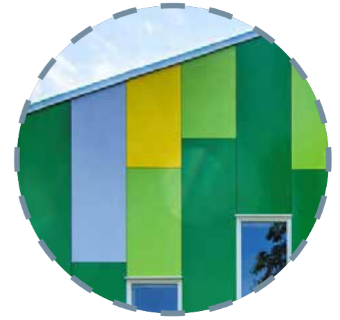
External Finish: Coloured Trespa Style Cladding Panels
