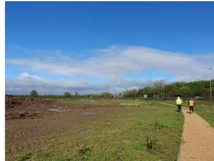
Site Photo A
